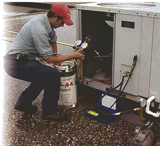
John O'Rourke, service tech from GT Air Systems in Kingston, Ontario services a rooftop unit.
