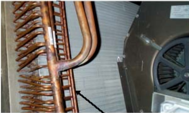
Liquid header and orifices
