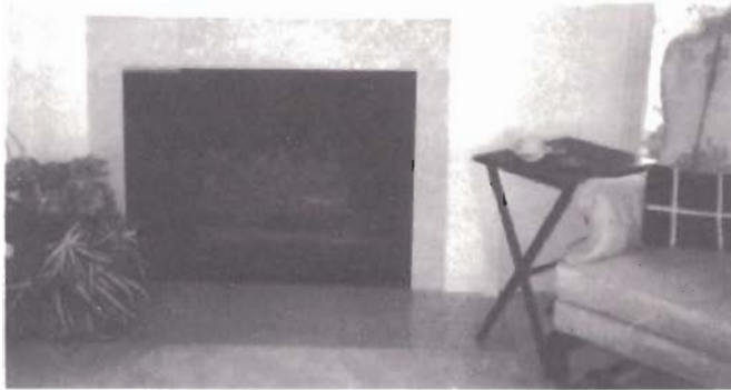
Gas log fireplaces like this one are a common source of soot in homes with ghosting problems.
